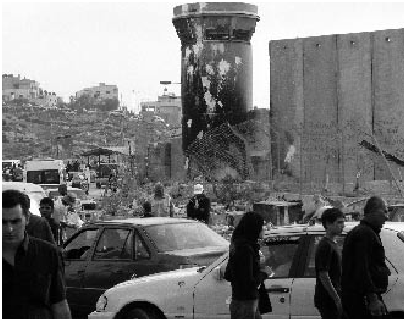
WATCHTOWER ALONG THE WALL AT QALANDIA CHECKPOINT, NORTH OF JERUSALEM. 27 OCTOBER 2004. PHOTO BY SAMIA HALABY.
